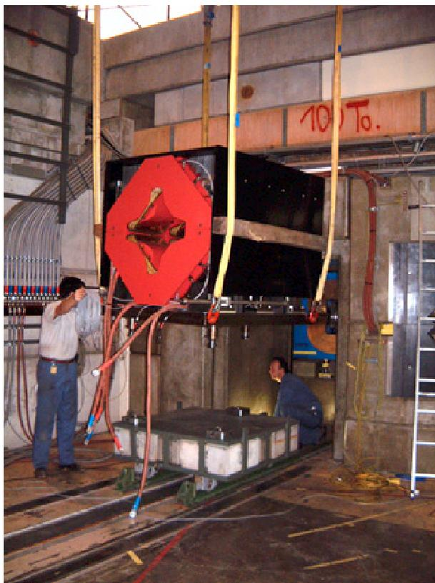
Figure 9: Photograph shows the triplet consisting of QSM-quadrupole magnets being lowered onto the the wagon designed to insert the elements into the "Z"-branch of the  $\pi$ E5 beamline.
